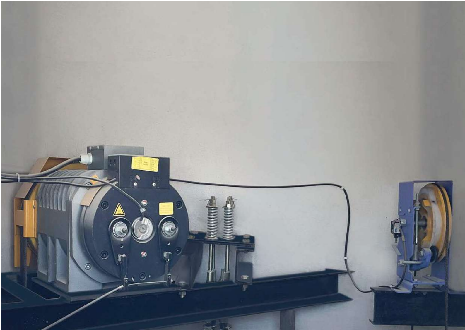
The machine of an MRL elevator is designed to fit in the elevator shaft
